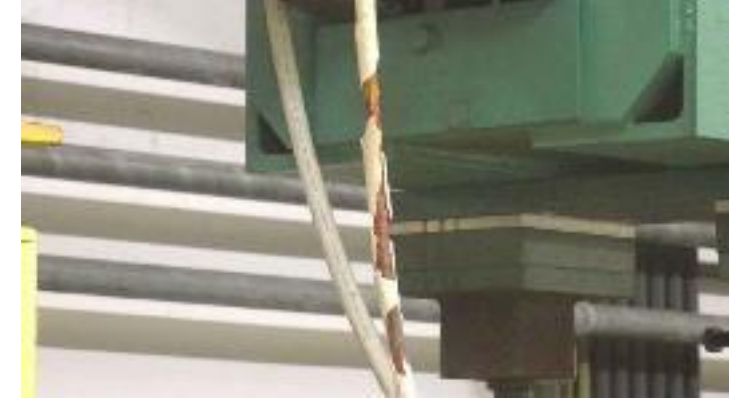
Cabling status inspection
