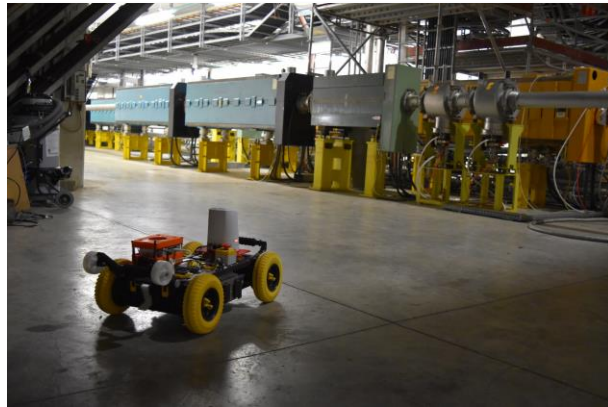
EXTRM robot (CERN controls)
