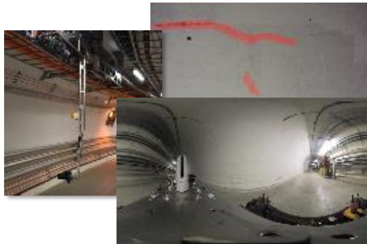
Tunnel structure monitoring
