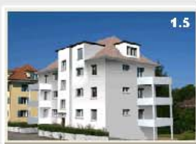
Steep roof attic
