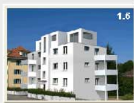
Flat roof attic
