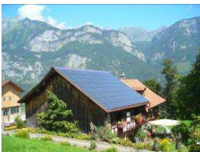
Links: konventionelle Integration (3-S, System Megaslate). Rechts: Integration neuartiger a-Si Module, entwickelt am Institute of Microengineering (IMT) der EPF Lausanne (Simulation).
