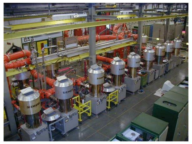
Figure 8: 200 MHz tetrode combination in operation at the CERN SPS since 1976 (Eric Montesinos).
