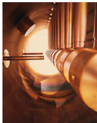
Drift Tube Linac 3 tanks
