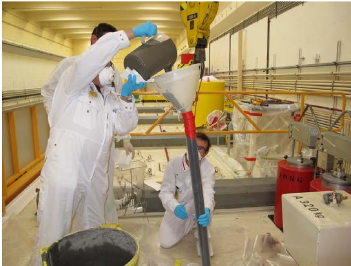
Cement filling from top of the cell
