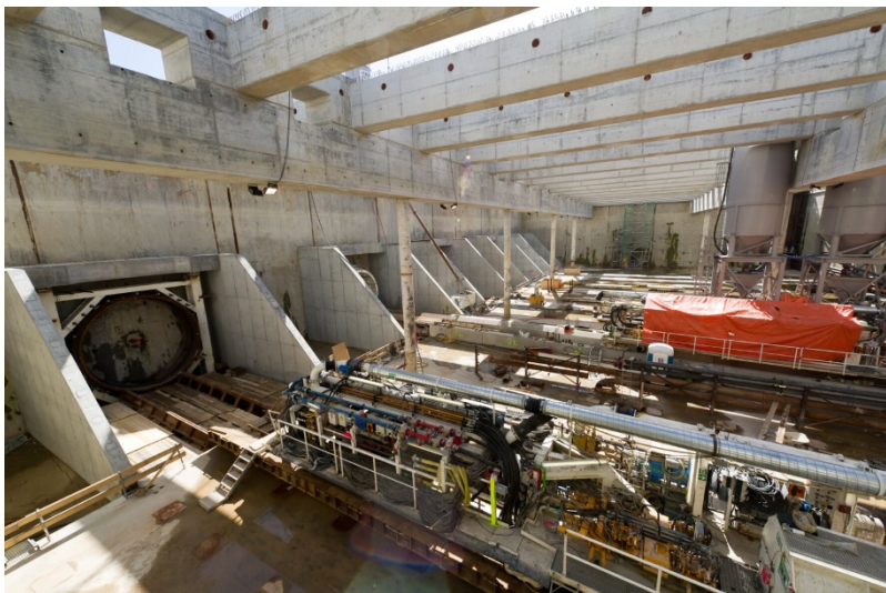
The building pit of the experimental hall, 10 April 2011
