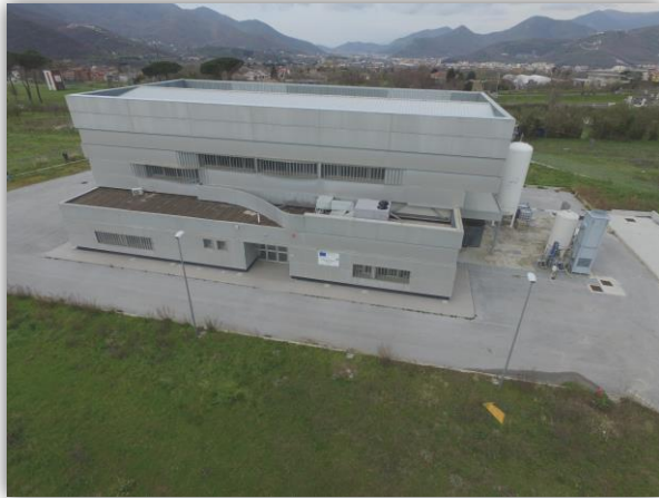
External view of the THor Test Facility
