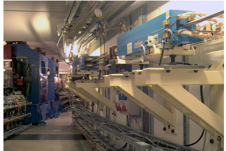
Booster mounted to inner tunnel wall
