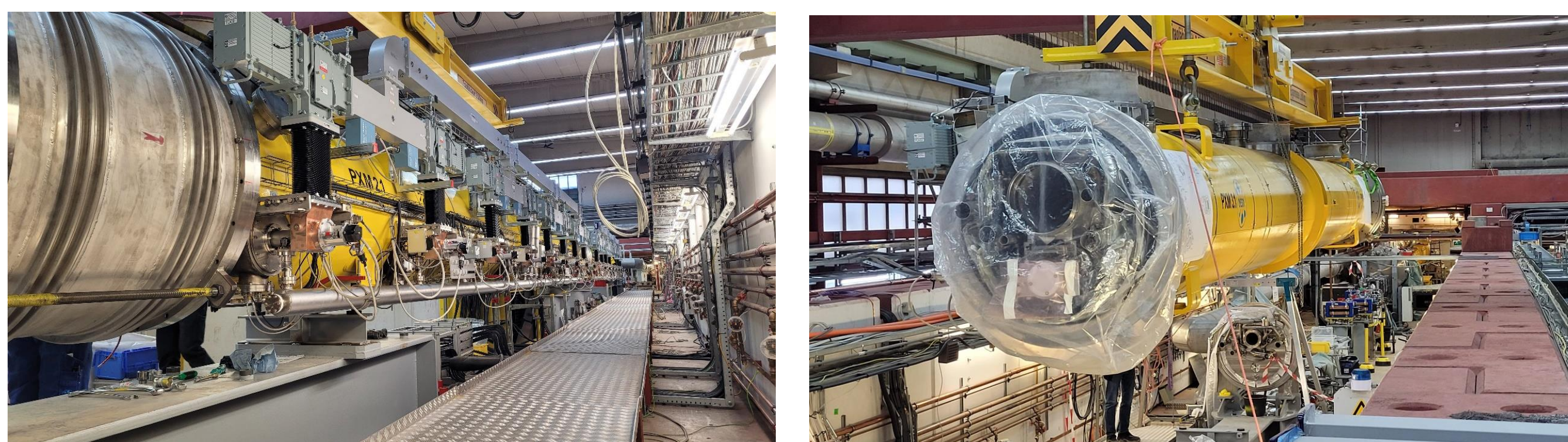
Installation of new CM for ACC2 and ACC3
