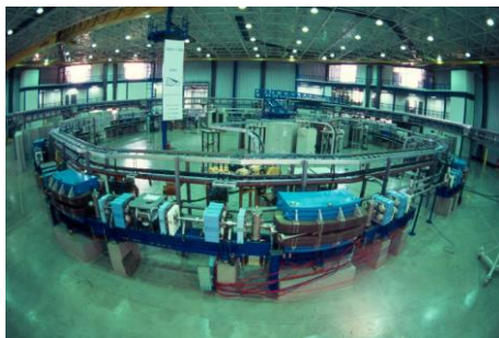
Assembly of ring concluded
