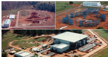
Construction of UVX at current CNPEM's site.
