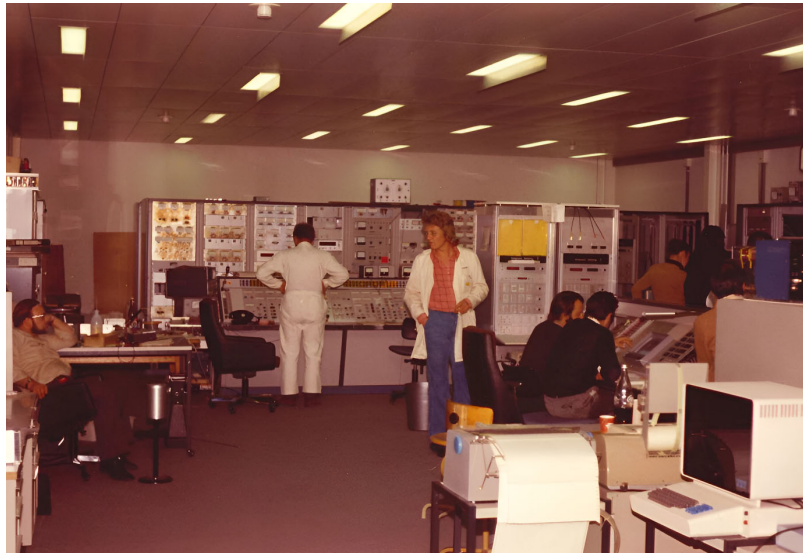
Original control room
