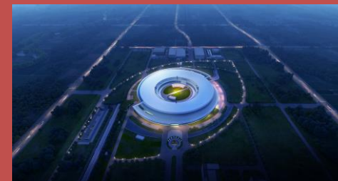
Hefei Advanced Light Facility
