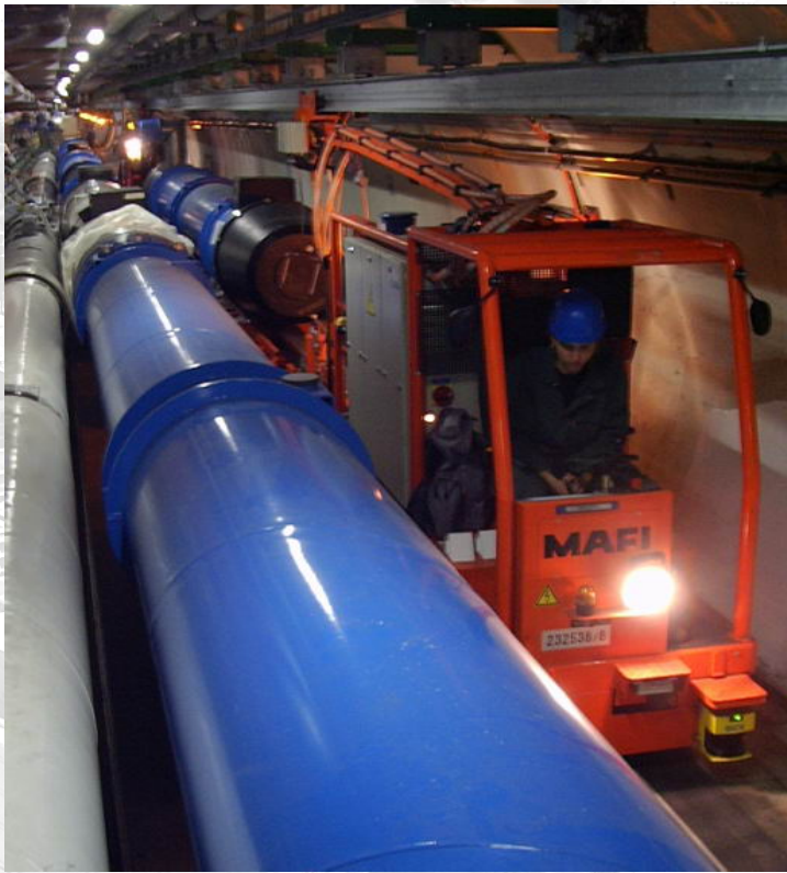
Custom-built vehicles transporting a 16m long, 33 tonne superconducting dipole along the LHC tunnel
